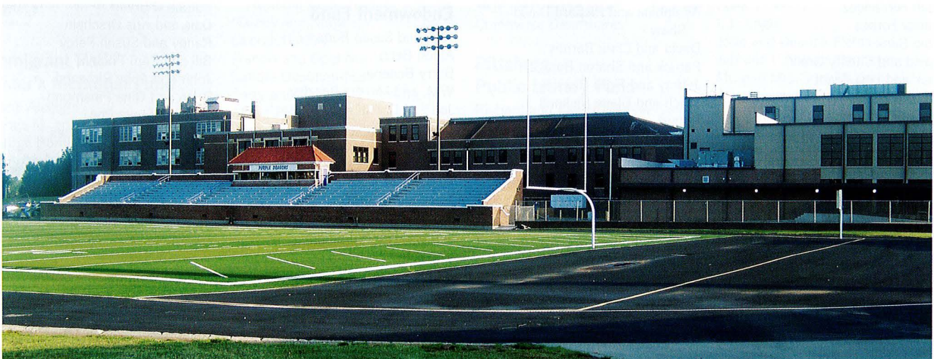
Improvements to Hutchinson Field were made possible through donations to the St. Mary's Colgan-USD 250 Facilities Improvement Task Force Fund.
