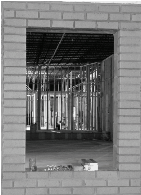
Plans are being made for a late August transition to the new Family Resource Center at 1600 N. Walnut.
